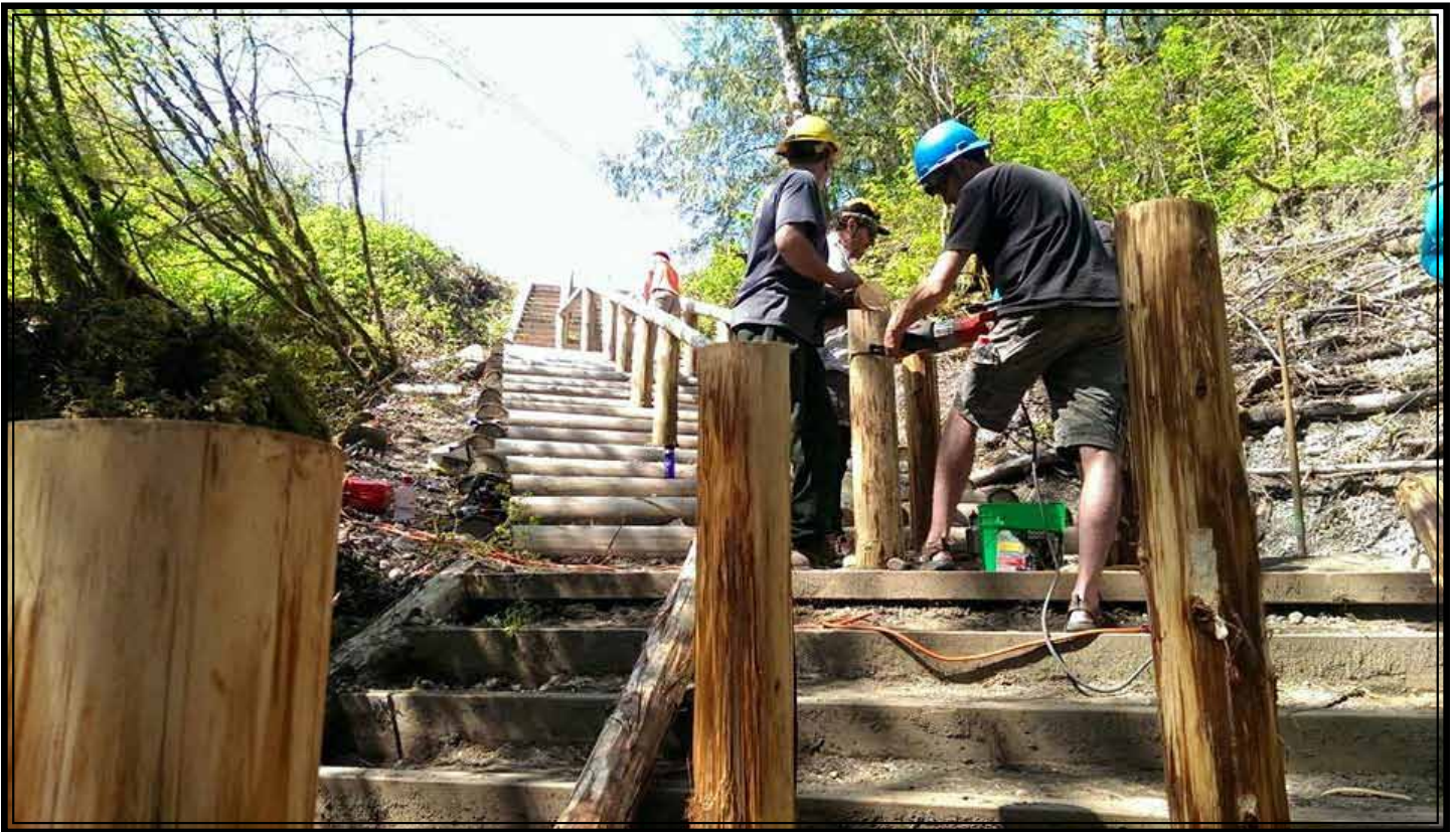
TOP: Cable Drop Access Party! Bottom: Setting and trimming posts for the boat slide rail. Photos Kim Filippini
